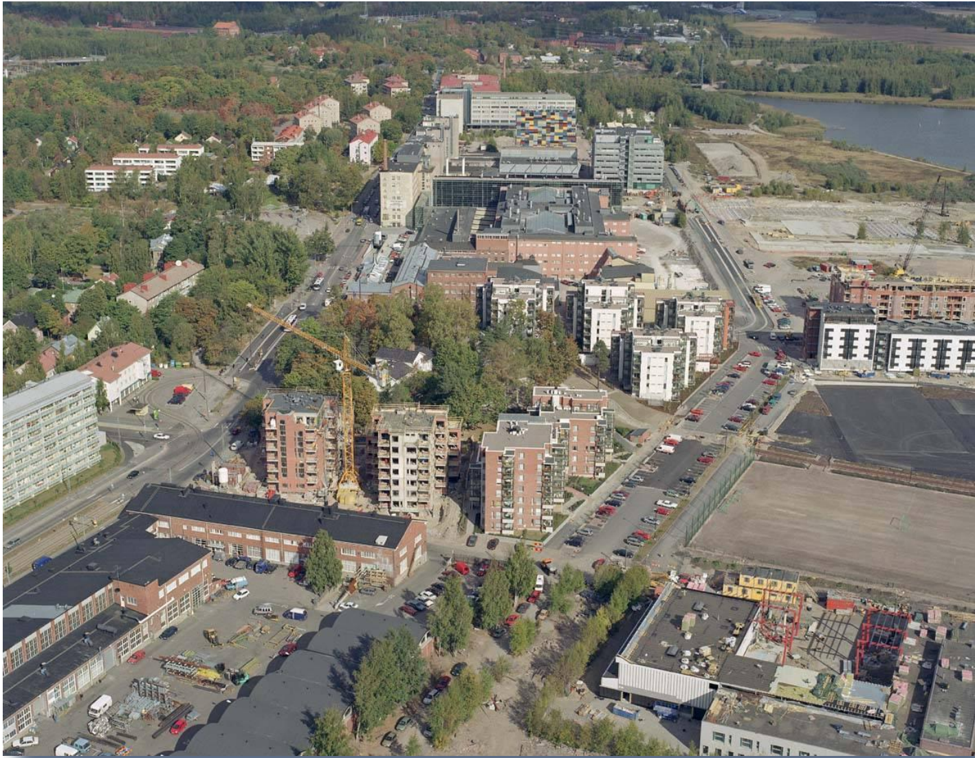
Construction work at Arabianranta
